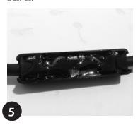
Fill rest of IP67 Slim J-Box with resin, ensuring that there are no large air gaps. Ensure resin is layered over bushings and into cover slots.
